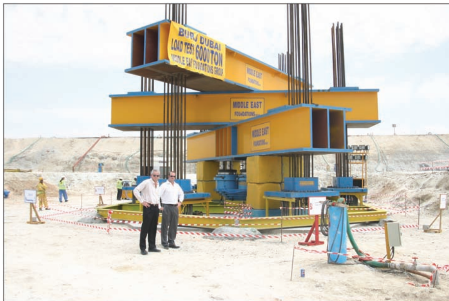
Fig. 7: Pile load test
