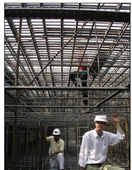
Fig. 8: Raft reinforcement
