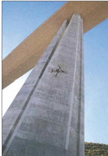
Fig. 3: Drone used for pier section inspection (Units: [-])
